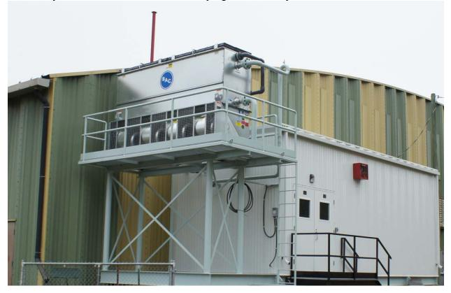
Dehumidifier has been installed, connections for electrical and to the curling rink have not been completed. The unit will be operated without the curling rink connection to assist with ice making at the start of the season.
