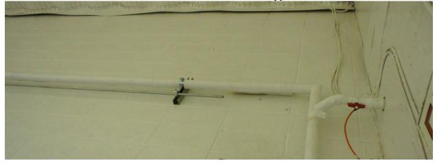
Brine connections to both rink ice slabs have been made pressure testing not completed.
