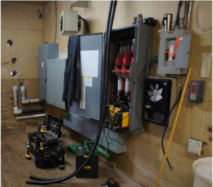
Electrical disconnects in plant building are not labelled correctly.
